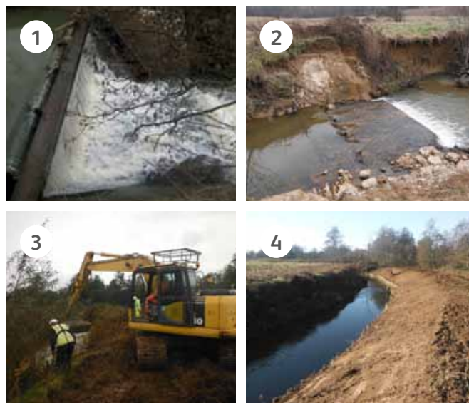
Clockwise: (1) Weir prior to works; (2) weir after wingwall / metal removal; (3) construction of gravel beds; (4) willow spilling protecting reprofiled right hand bank.
